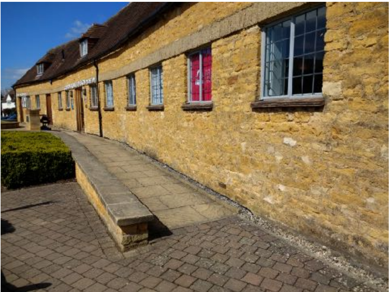
The Museum entrance, via a ramp from Russell Square
